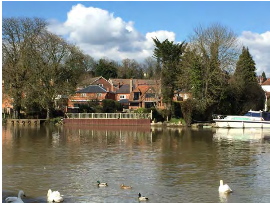
Steel piling of the river bank
