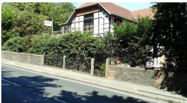
Railings replacing flint walls, St Peters Hill
